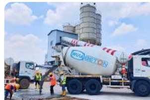
Pengecoran Beton Ready Mix Ready Mix Concrete Casting
