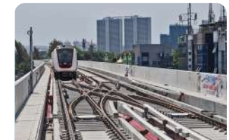
Sistem Perkeretaapian Railway Systems
